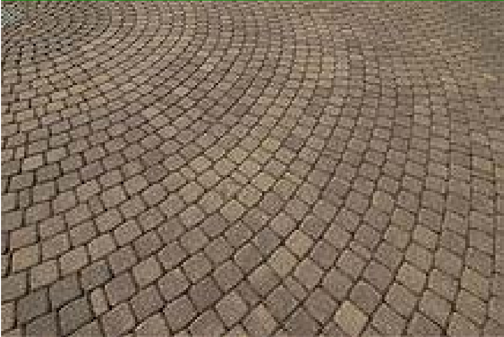
Concrete paver blocks in a circular pattern
