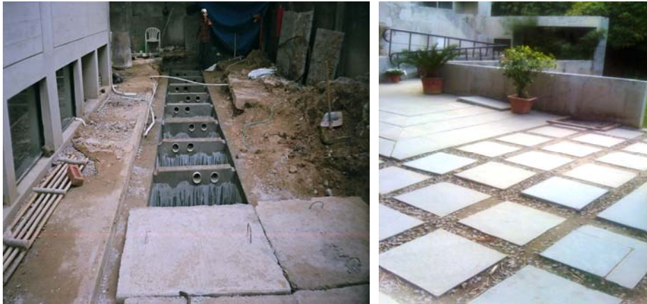
Photo 04: Rain-Water Harvesting Pit in AAGC and Paving Techniques
