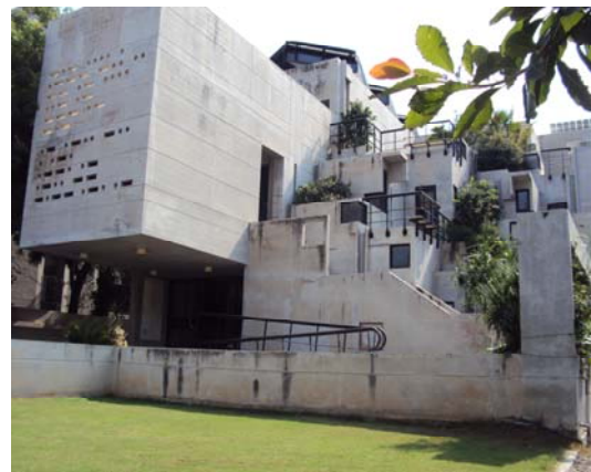
Figure 02: Building Massing for Effective use of Day-lighting through Orientation
