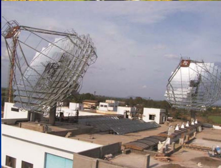
A Solar Steam Generating System at Global Hospital, Mount Abu, Rajasthan
