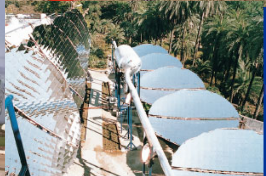
A Solar Steam Generating System at Global Hospital, Mount Abu, Rajasthan
