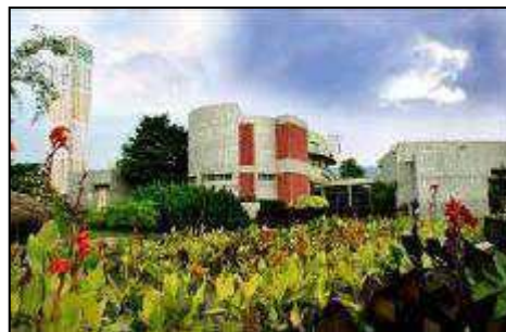
Root Zone Treatment System
