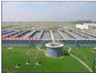
On-site Waste Water Treatment Plant
