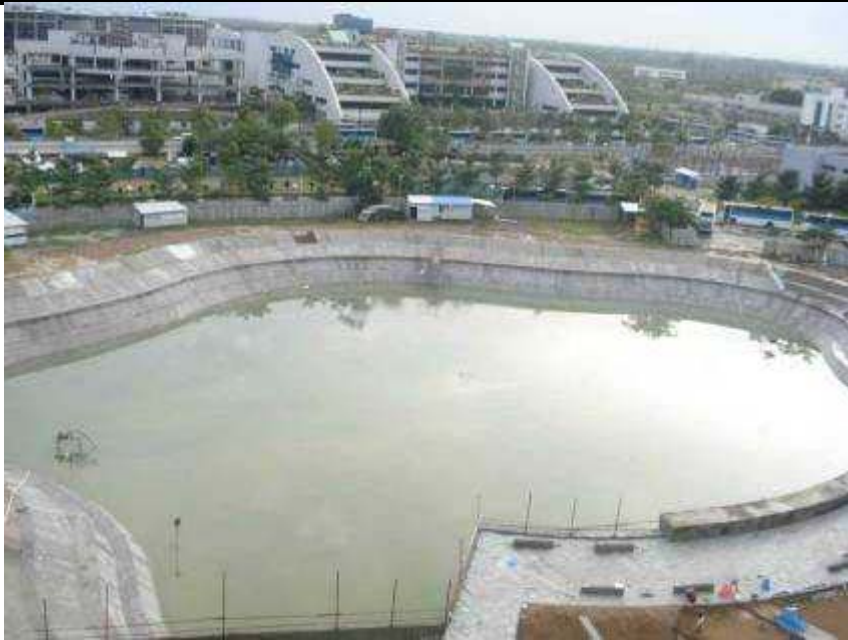
88953 m3 capacity storage pond
