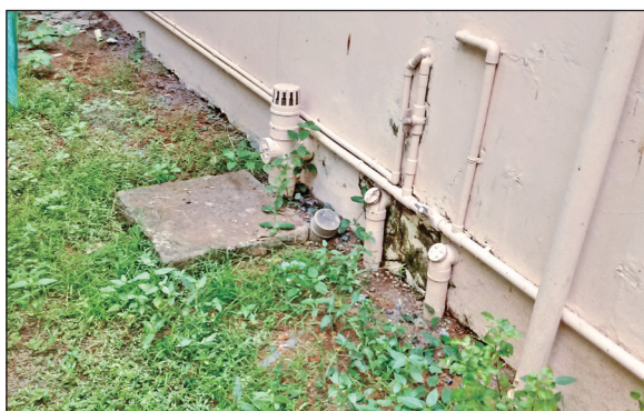
Photo 4: Grey water connected to a separately constructed soak pit
