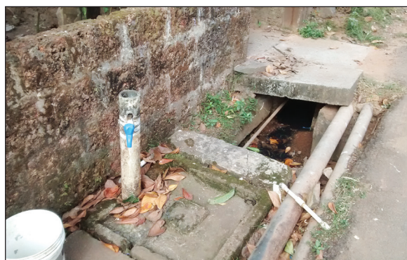
Photo 5: Grey water flowing into the open drain.
