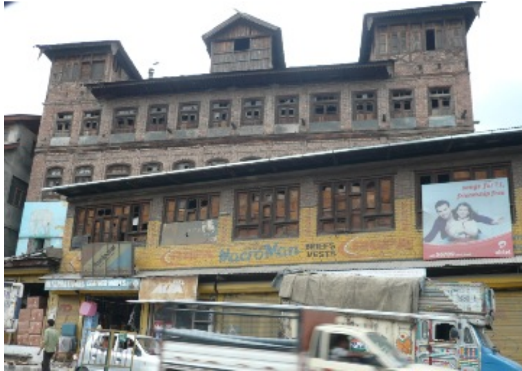
An old Kashmiri four/five story house built in Taq system stands tall in the background of some new constructions in a Srinagar market
