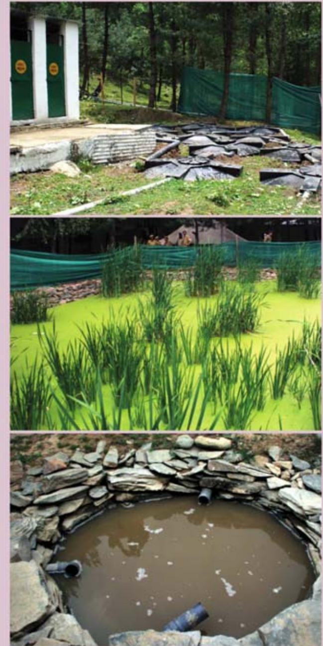
Cleaning the waste of millions: toilets are dosed with microbes and so don't smell; waste goes to a reed bed and oxidation tank.
