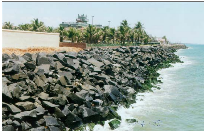
Figure 3: Artificial sea wall built along the Marina beach
