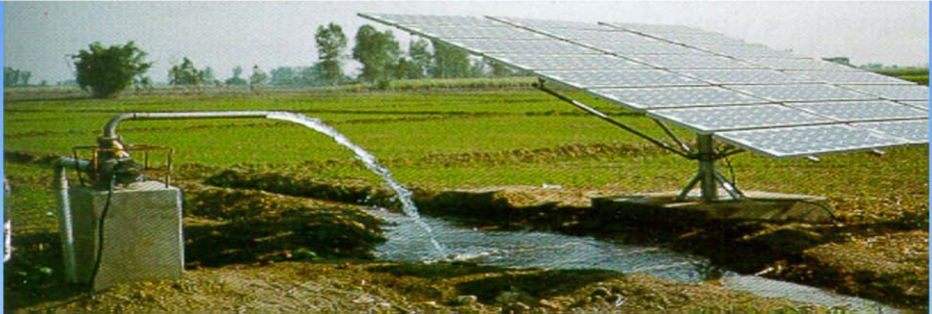
SPV Water Pumping System at a agricultural farm in Punjab
