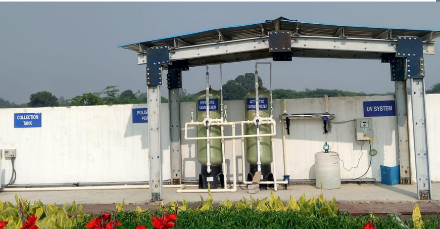
Tertiary treatment by UV treatment and activated carbon filter
