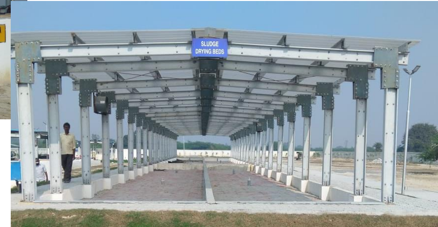
Drying beds covered by polycarbonate sheets
