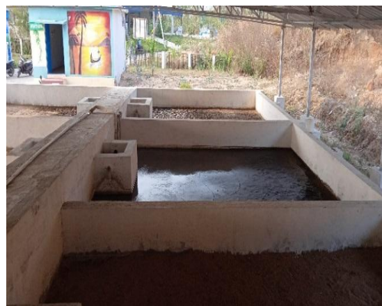
Figure 8: Sludge drying bed in FSTP (Source: Vandana/CSE, 2020)
