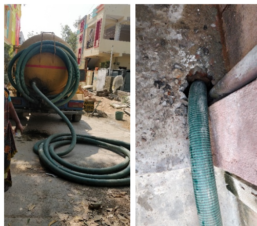
Figure 7: Emptying process captured of a twin pit system (Source: Vandana/CSE, 2020)
