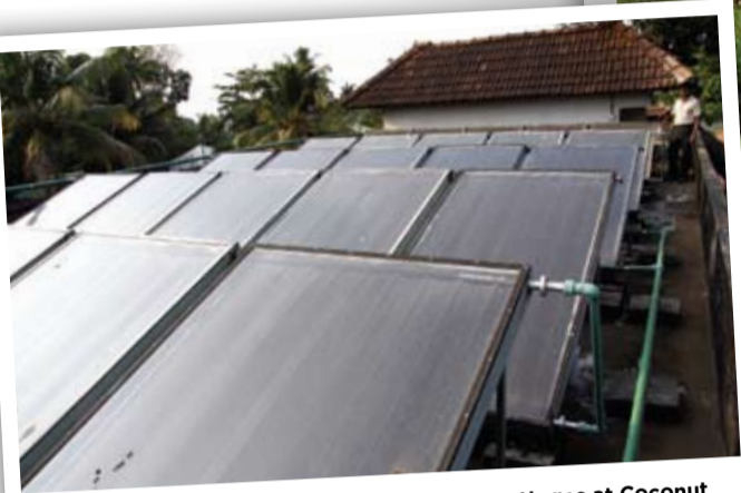
Solar panels for heating water for the entire cottages at Coconut Lagoon
