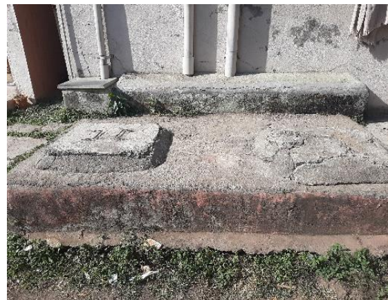
Figure 4: Direct connection to sewer line in Satpur Gaon (Ekta/CSE, 2020)
