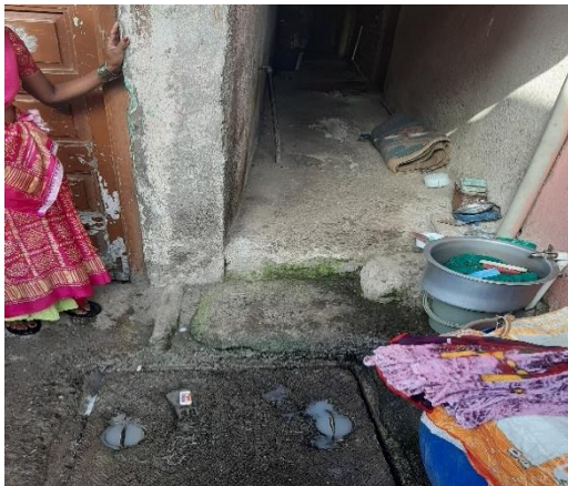
Figure 3: Direct connection to sewer line in Satpur Gaon (Ekta/CSE, 2020)
