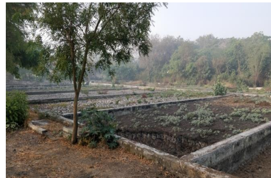
Figure 5: Sludge drying beds at STPs (Source: Mudit/CSE, 2020)
