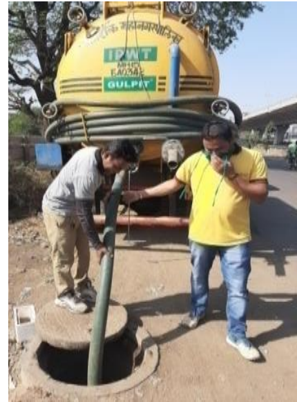
Figure 6: Discharge by vacuum truck in trunk sewer (Source: Ekta/CSE, 2020)
