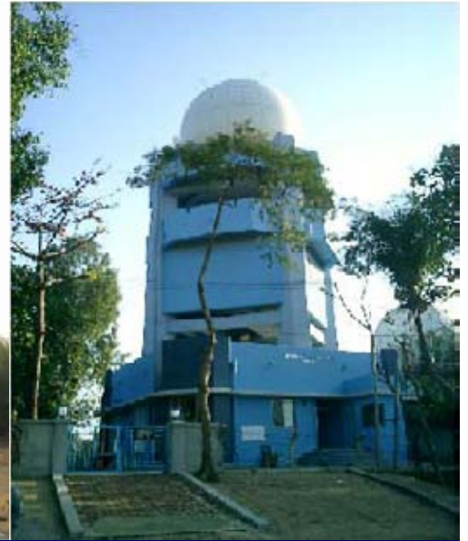
Cox's Bazar Radar
