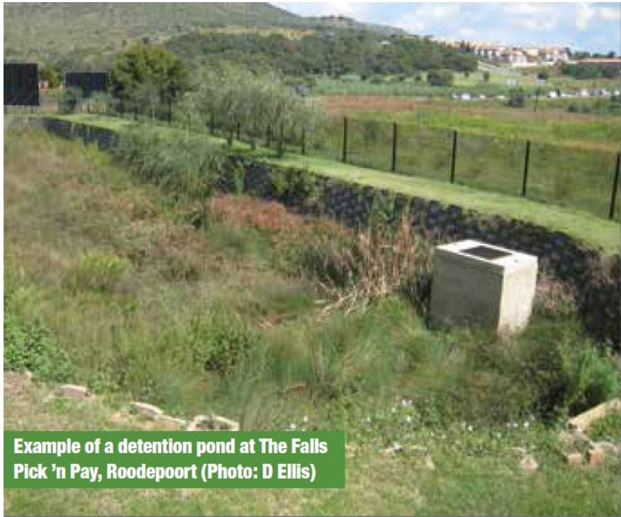
Bio-swales collect and treat stormwater from The Falls Pick 'n Pay parking area for later use as irrigation water (Photo: D Ellis)
