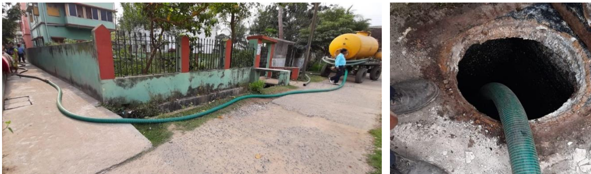
Figure 5: Emptying Process through vacuum tanker, source: Manish/CSE, 2020
