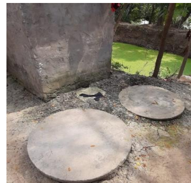
Figure 4: Twin - Pit system, Source: Manish/CSE, 2020
