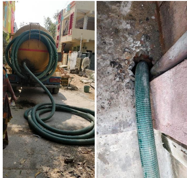
Figure 6: Emptying process captured of a twin pit system (Source: Vandana/CSE, 2020)
