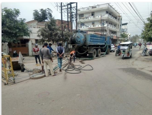
Jetting Machine Cleaning the Sewer Line
