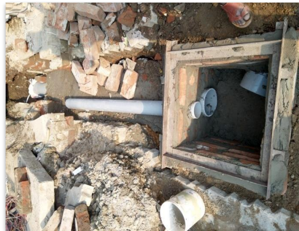
HH being connected to sewer chamber
