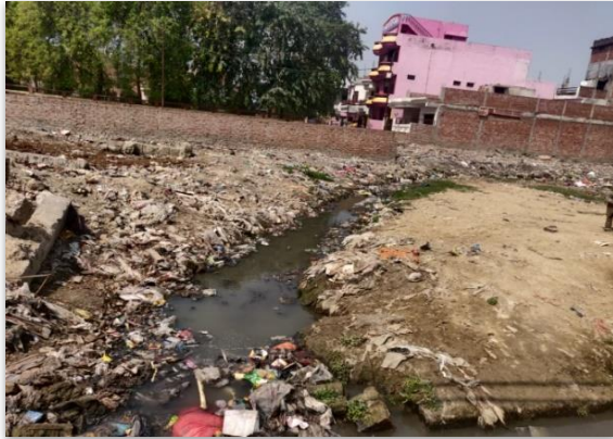
Open drain ending at open ground
