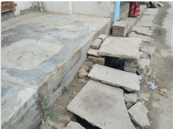
Septic Tank of a Household
