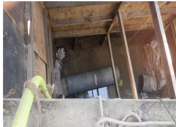
Under Construction Sewer System
