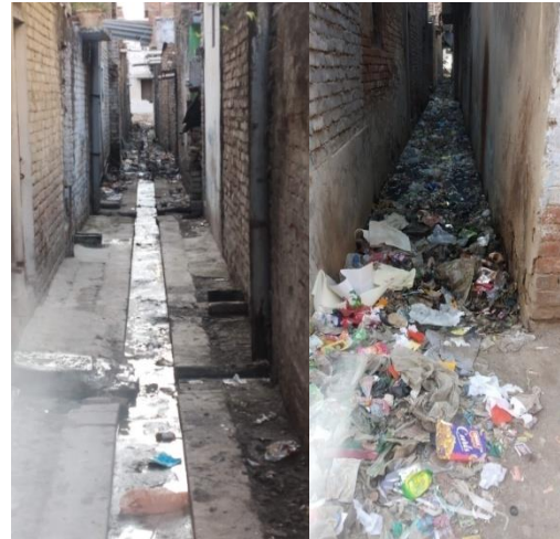
Containment emptying at open Drain
