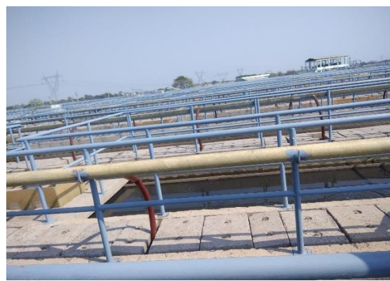
UASB reactors
