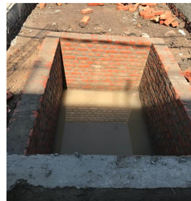
Figure 3: Fully Lined tank under construction (Source: Harsh/CSE 2020)
