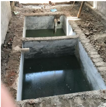
Figure 5: Septic tank under construction (Source: Harsh/CSE 2020)
