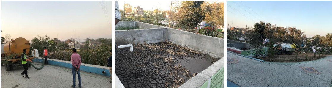
Figure 10: Emptied FS is disposed at FSTP Bijoli, Jhansi (Harsh/CSE, 2020)
