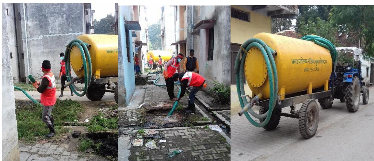
Figure 3: Mechanical emptying in process (on left) and tractor mounted vacuum tanker (on right) (Manish/CSE, 2020)
