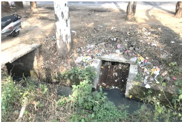
Figure 2: Open Drain tapped at Barrage Road (Harsh/CSE, 2020)
