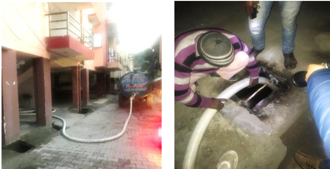
Figure 6: Emptying process captured near Palika Chowk in a common septic tank tank of 8 households. (Harsh/CSE, 2020)
