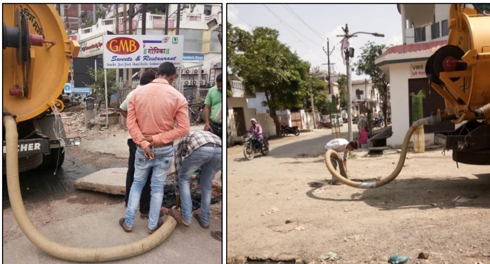
Figure 3: Cleaning of choked sewer by government emptier
