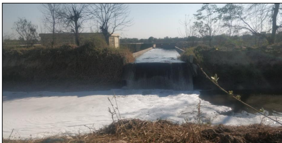
Figure 6: Treated wastewater discharging from an STP
