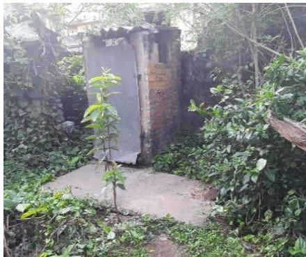
Figure 3: Fully Lined Tank (Source: CSE 2020)
