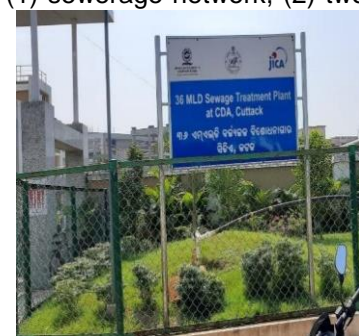
Figure 2: Sewage Treatment Plant (Source: CSE, 2020)
