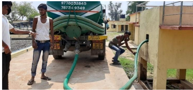
Figure 8: Septage Treatment Plant (Source: CSE, 2020)
