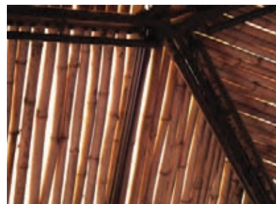
Bamboo roof as viewed from inside the eco-huts
