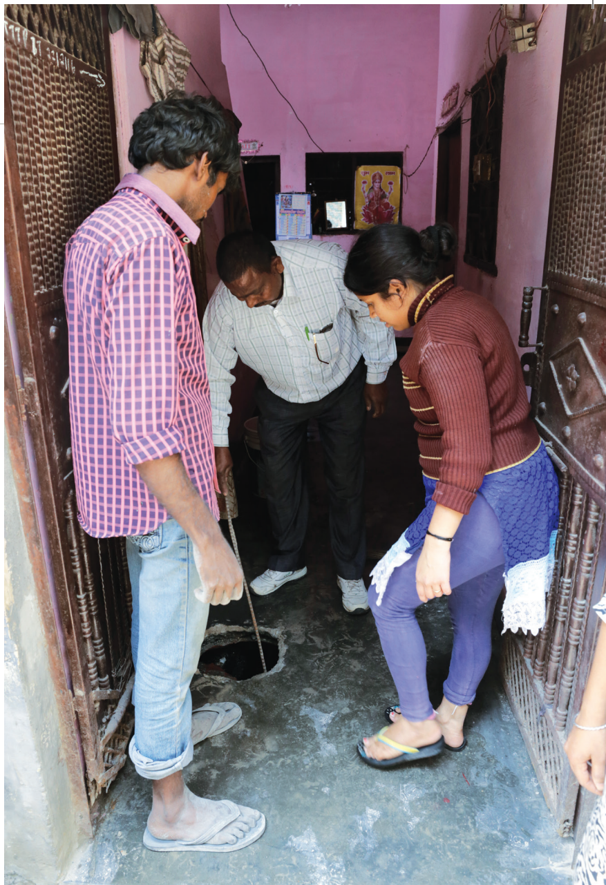
This family at Balram Nagar in Loni, Ghaziabad, has a big, partitioned septic tank but its effluent is discharged into an open drain
