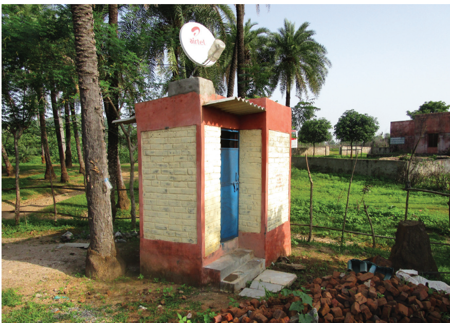
ECOSAN toilets in village Danodhar
