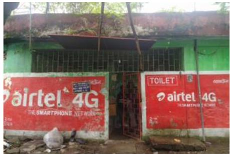
Figure 6: Public Toilet in Ward no. 10 (Vikash/CSE/2020)
