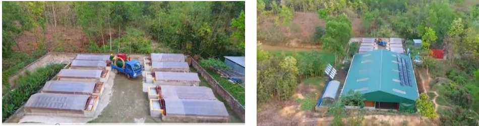
Figure 5: Sakhipur Faecal Sludge Treatment Plant (Co-compost plant)
