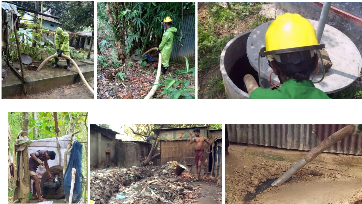
Figure 3: Septic tanks and pit emptying (mechanically and manually) in Sakhipur
