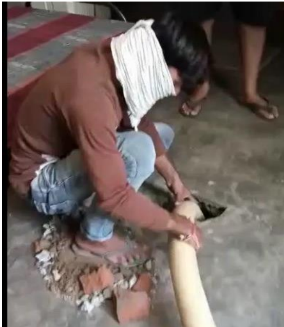
Figure 5 : Emptying in process by mechanical means (Harsh/CSE/2020)
