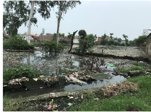
Figure 2: Open Drains overflowing in to low lying areas/open fields. (Harsh/CSE/2020)
