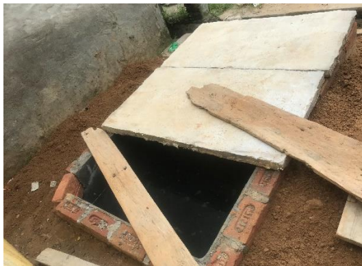
Figure 3: A septic tank under construction. (Harsh/CSE/2020)
