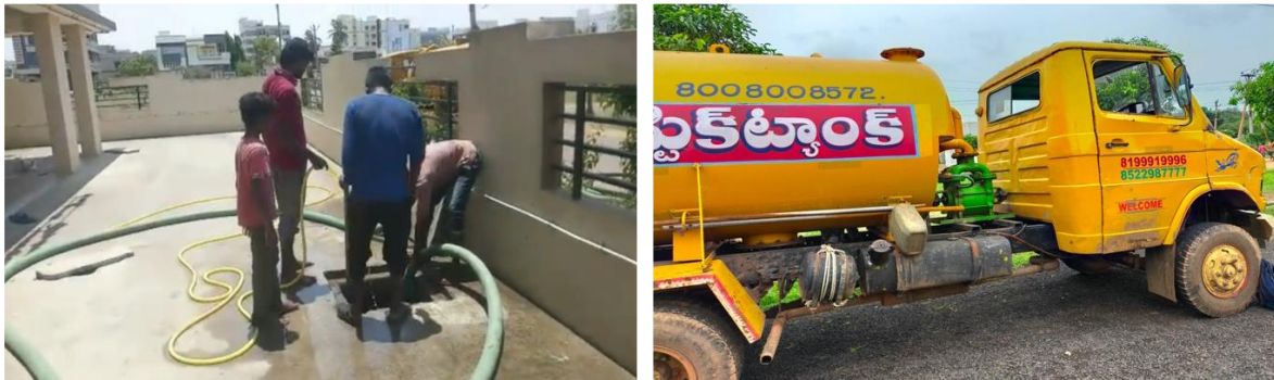
Figure 3: Emptying process in household through private truck mounted vacuum tanker
