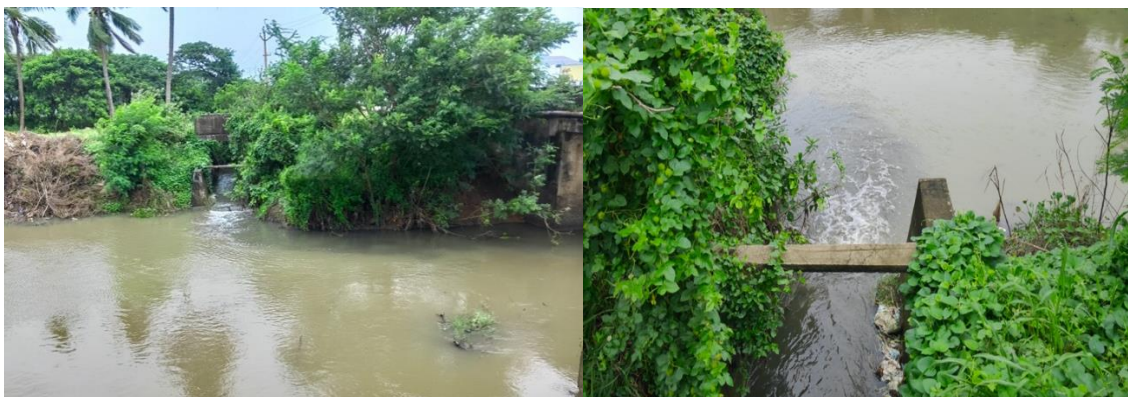
Figure 5: Storm water drains ending up in the drainage canal near Mandapeta- Alamuru road
