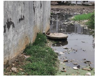
Figure 4: CT's tank connected to open water body (Abhishek/CSE, 2020)
