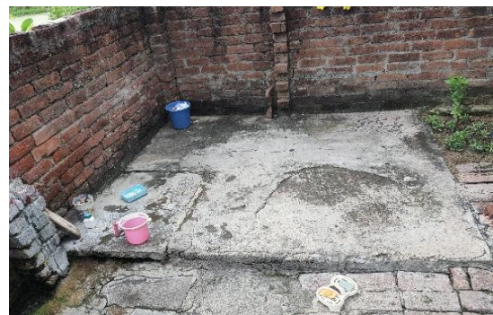
Figure 3: Square shape FLT found in Barkhedwa ward with 2 chambers
