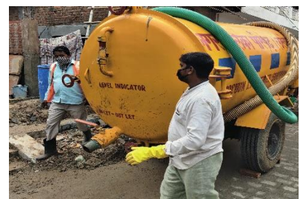
Figure 5: Desludging by vacuum tanker in Santosh Nagar (Source: Abhishek/CSE, 2020)
