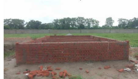
Figure 7: FSTP, under construction (Source: Abhishek/CSE, 2020)
