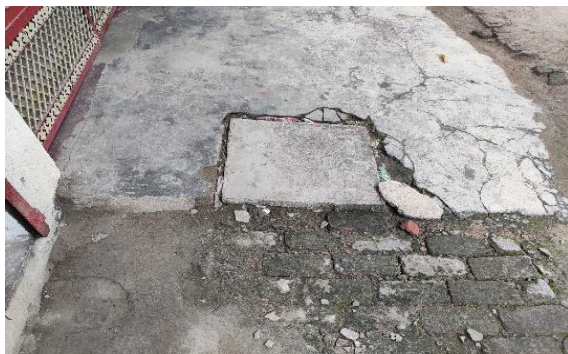
Figure 2: ST with 2 chambers found in Shiv Colony, half of which is inside the house and half is outside for emptying (Abhishek/CSE, 2020)
