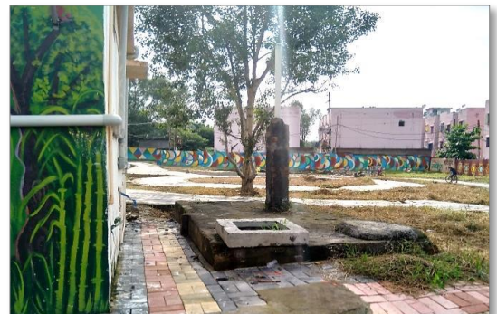
Figure 1: Septic tank of a public toilet near Lalbagh
