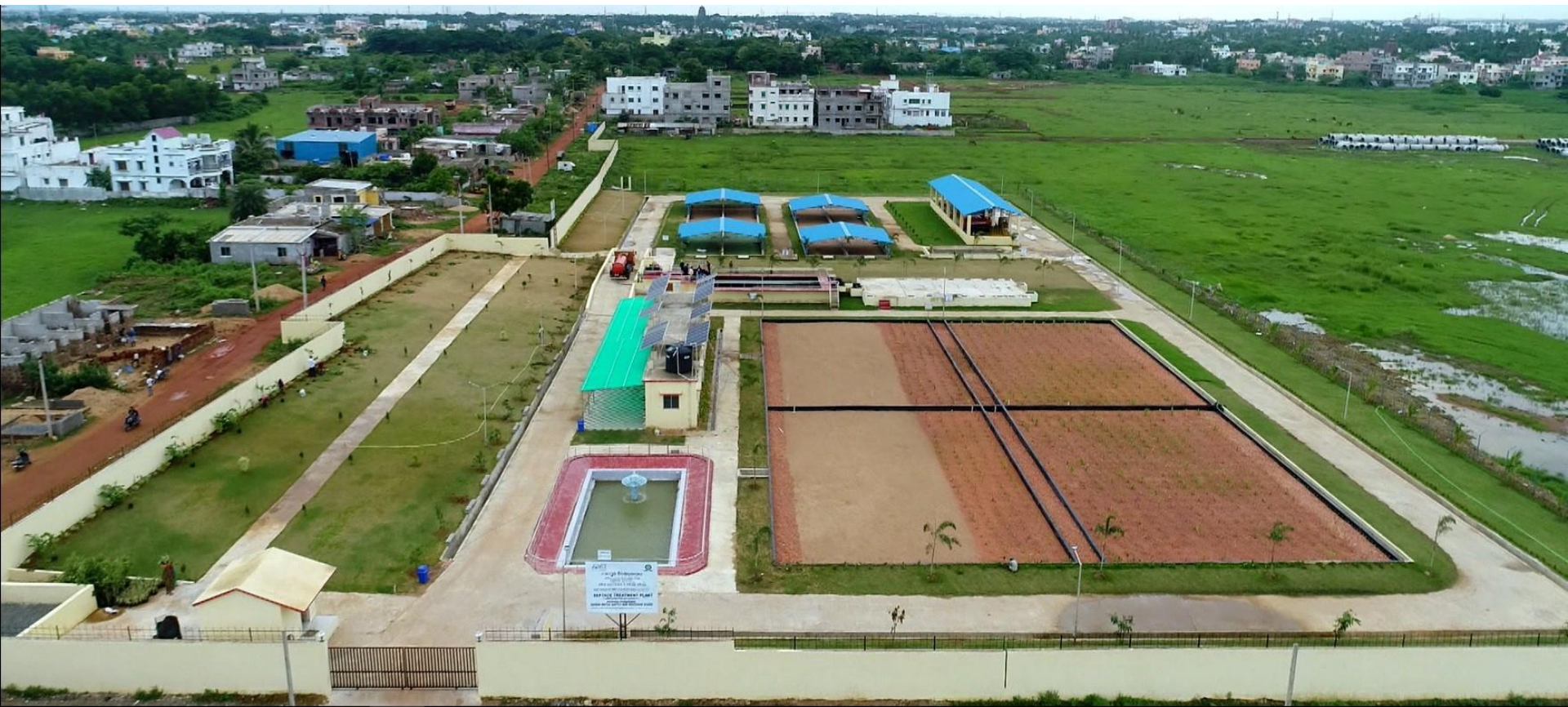
Photo: Bhubaneswar Septage Treatment Plant
