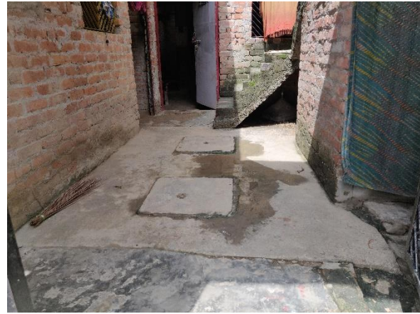
Figure 2: 2 chambered septic tank
