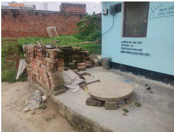
Figure 3: Septic Tank constructed under PMAY
