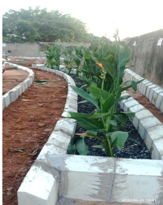
Lane Level: Hybrid leach pit and absorption trenches
