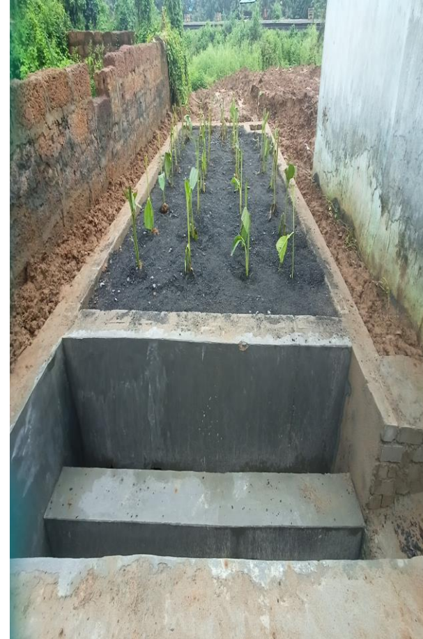
Community Level: Construction wetland/waste stabilisation pond
