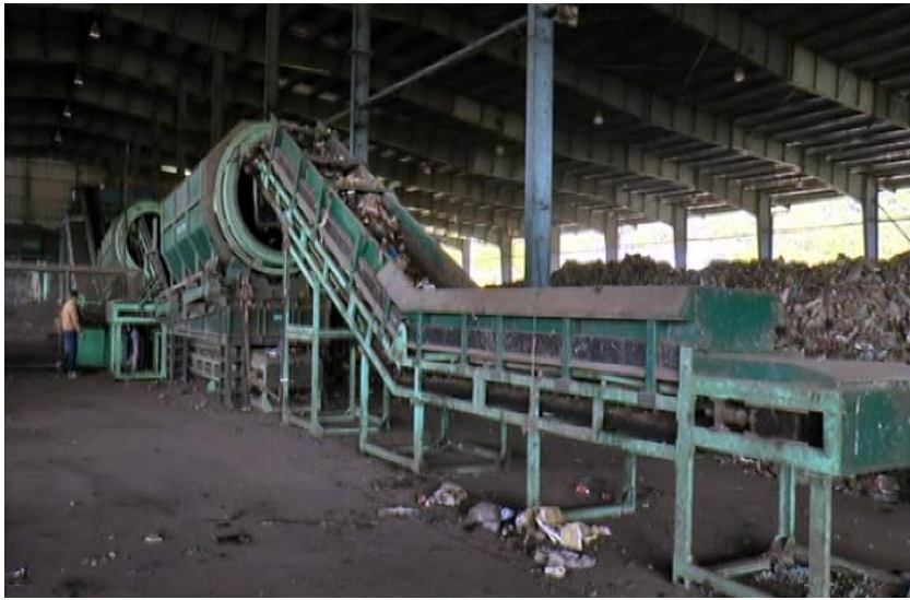
Lamdeng Waste to Compost Plant
