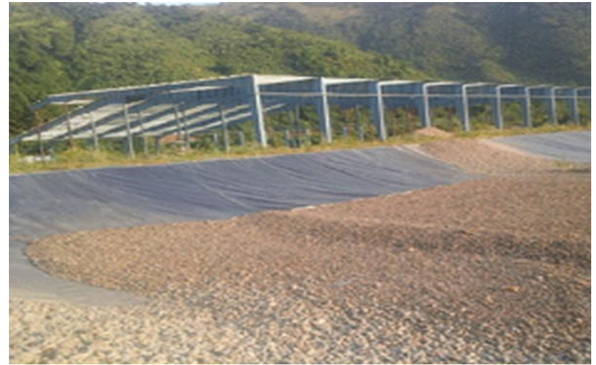
Sanitary Landfill at Lamdeng
