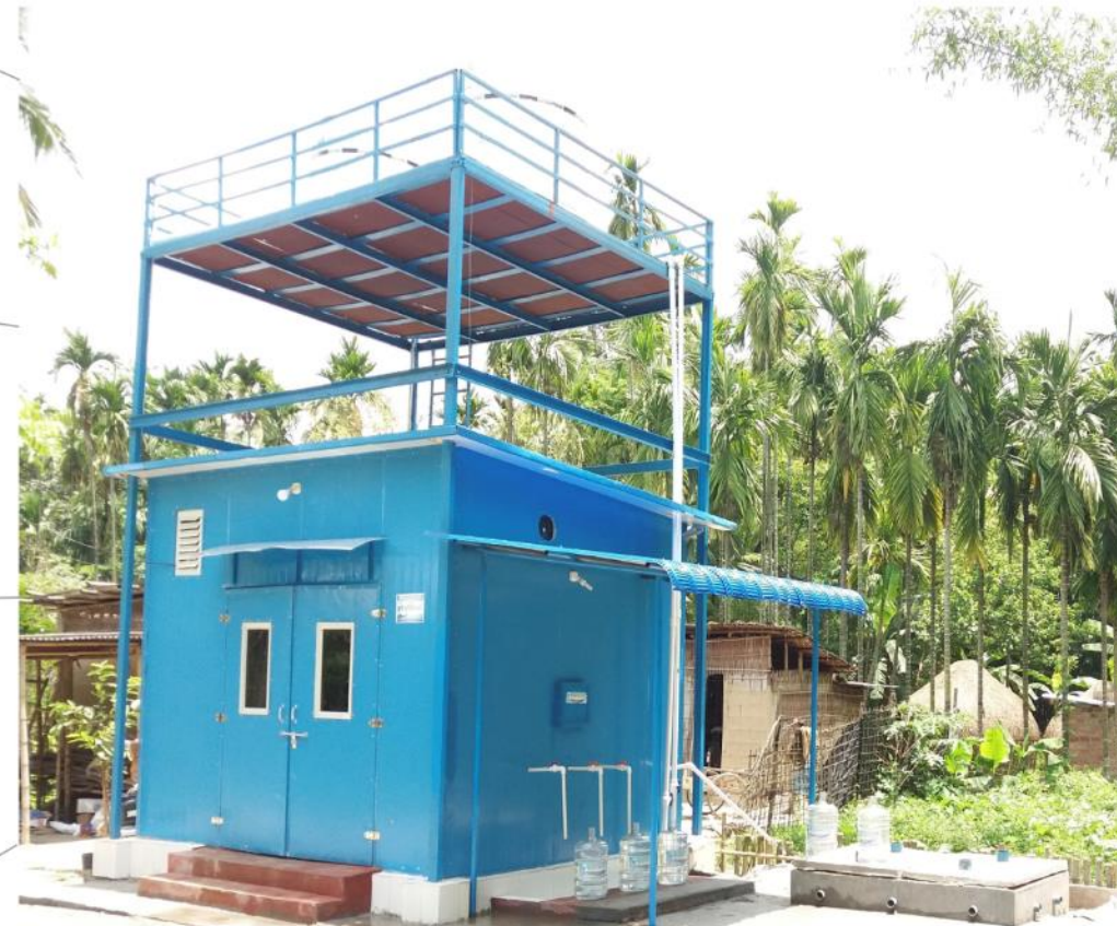
1,000 Liter Per Hour Arsenic Removal System in Nalbari, Assam financed by Tata Trusts
