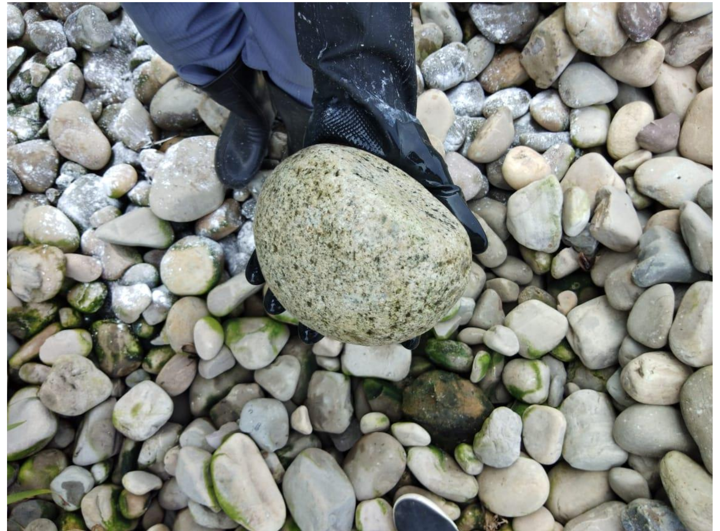
AFTER CLEANING: Algae growth scrubbed off from PGF stones
