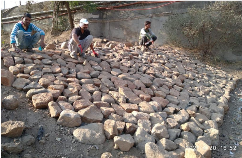
Pitching and barricading along the river
