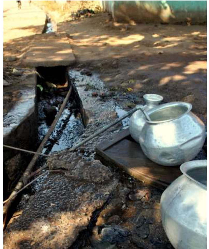
Drinking water situation in rural Keonjhar district, Odisha; CSE 2017
