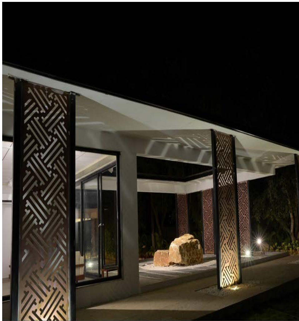
The close-up view of the north-east corner. The columns (thirty six in total) not only support the roof but also act as ornamental architectural elements.
