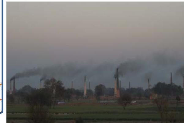
Firing Technology - Fixed Chimney Bulls Trench Kilns 75% of production of India (30,000 – 40,000 brick kilns in India) Coal (80%) & Biomass (20%)
