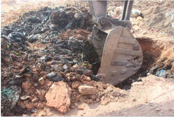
Pit Excavation for Geo Technical investigation in progress.
