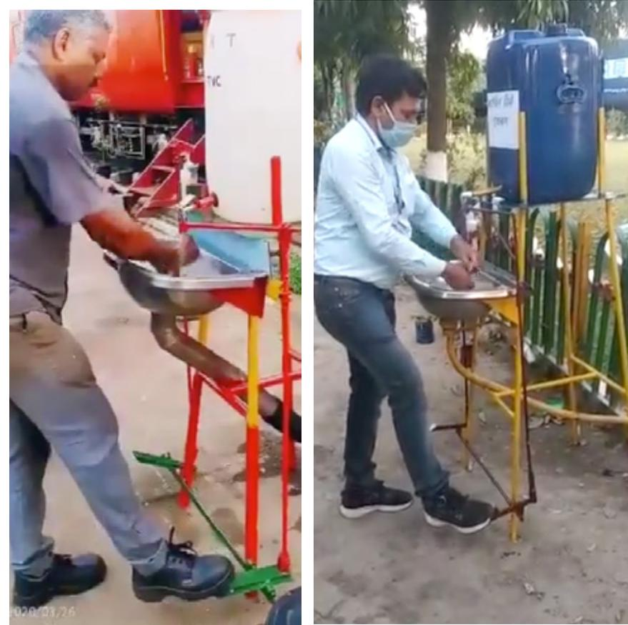
Foot operated Iron bars can be fitted on a tap to create a motion of pushing inside to open the valve
