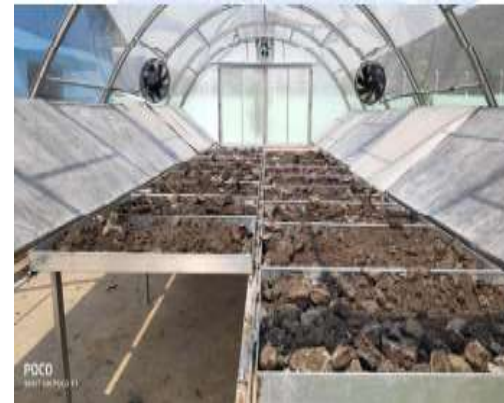
6. Sludge Pasteurization Unit
