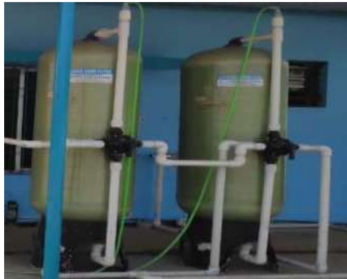
5. Activated Carbon Filter
