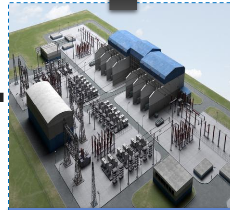
Generating Stations (containing equipment such as Transformers, Reactors, Generating Units, Buses, Breakers, Isolators, etc.)
