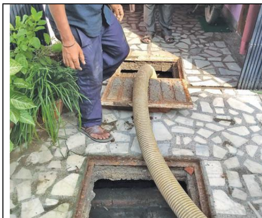
Septic Tanks need to be regularly emptied with proper safety gear.
