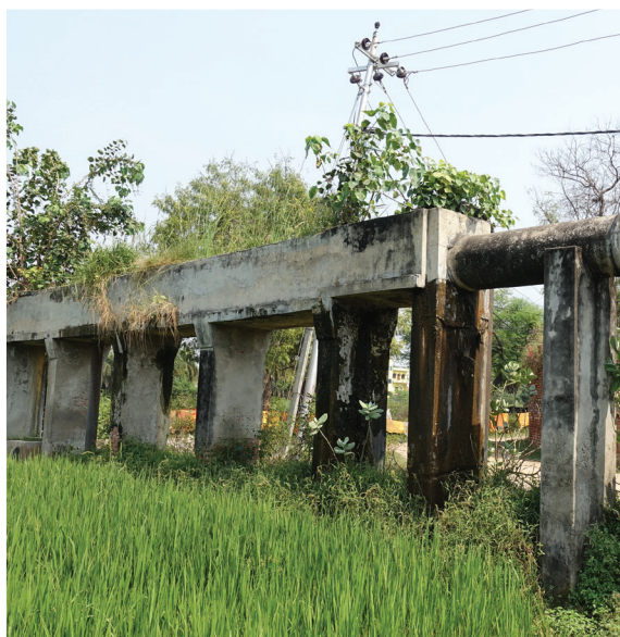
Mixing tank of sewage & tubewell water
