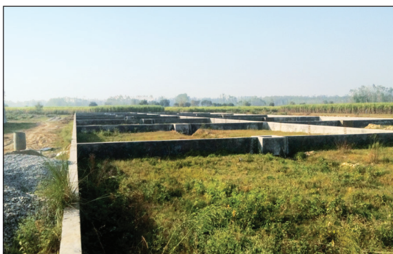
Figure 6: 24 MLD UASB+Aeration Sewage Treatment Plant (under construction).
